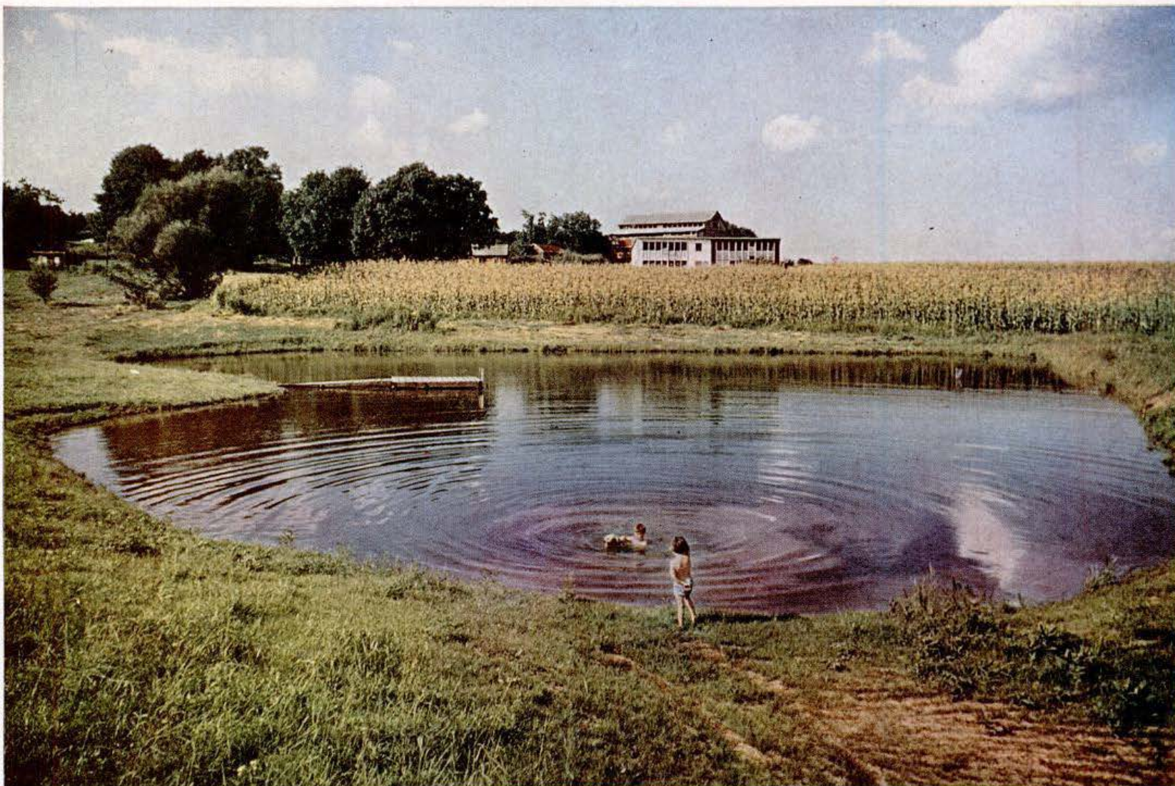
CHICKEN FARM POND fed by rain water cost $850, was built as a year-round supplementary source of water for crops and chickens and also as a fire protection.
